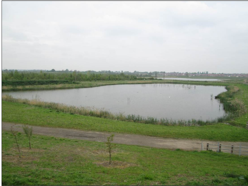
Photo 5 Large attenuation pond AP2 for the A421 improvement scheme
