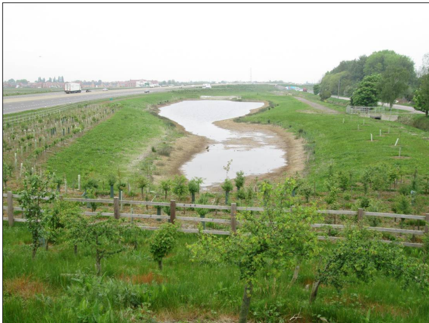
Photo 4 Attenuation pond AP1 for the A421 improvement scheme
